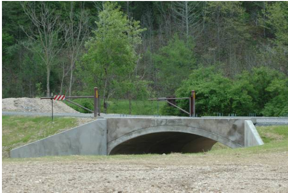
A side view of the new Turkey Bay bridge.
