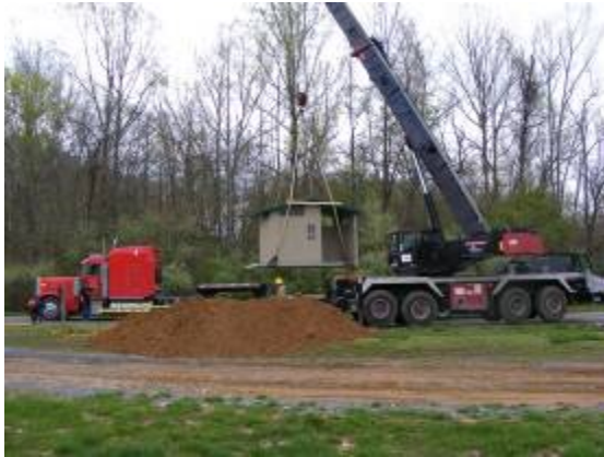
The new SST being installed at Turkey Bay.
