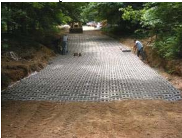
A hardened creek crossing designed for sustainability.
